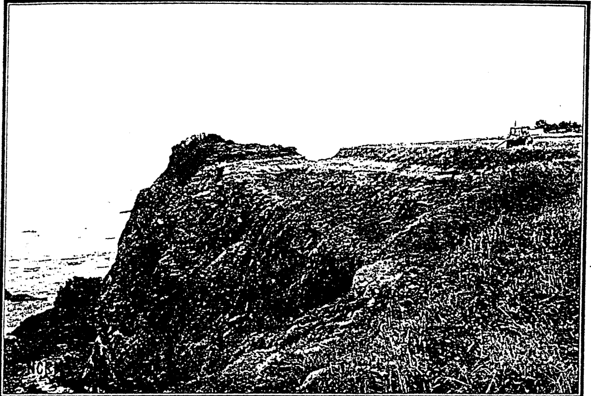
Photo #1: Overview of RR grade from cliff approximately midway between Site-02 and Isolate-01, viewing north-northwest. Note cutbank through bluff to avoid protruding point in cliff and the heavily eroded channel that has removed much of the grade.
