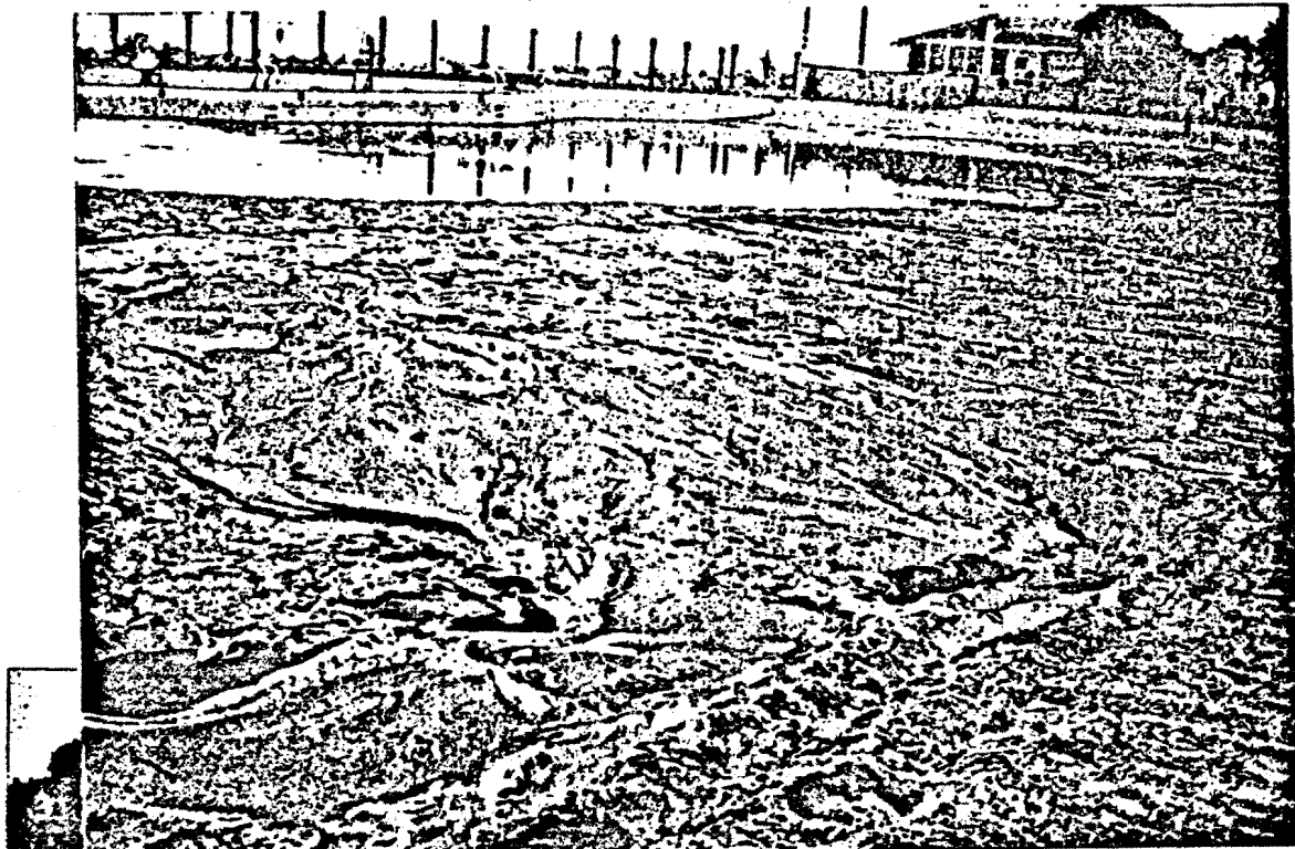
Above: Sand boils formed in Redondo Beach Seaside Lagoon beach area from liquification
