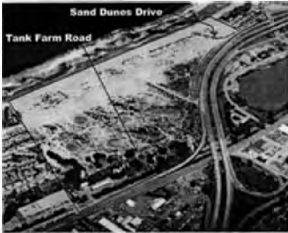
Figure 1. Oblique Aerial View of Project Site Illustrating Project Boundaries and Existing Paved Roads.
