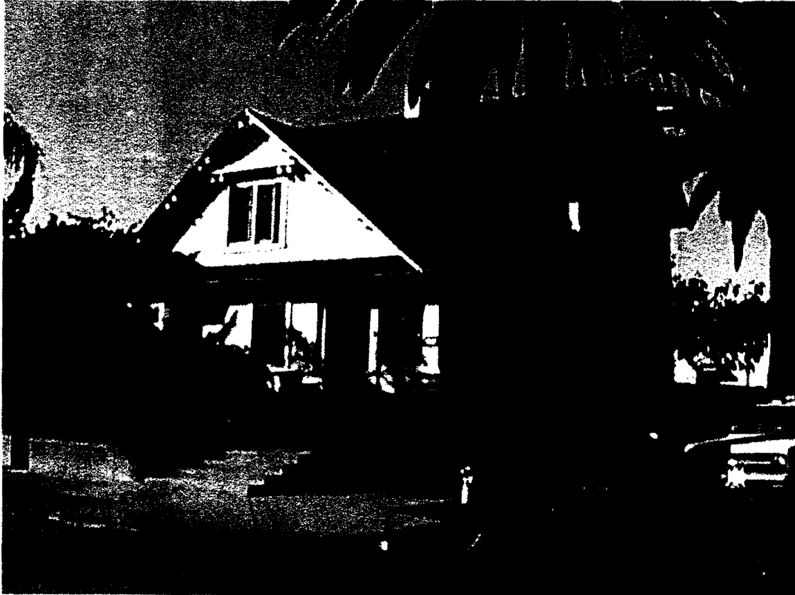
View of front and North side from Electric Avenue
