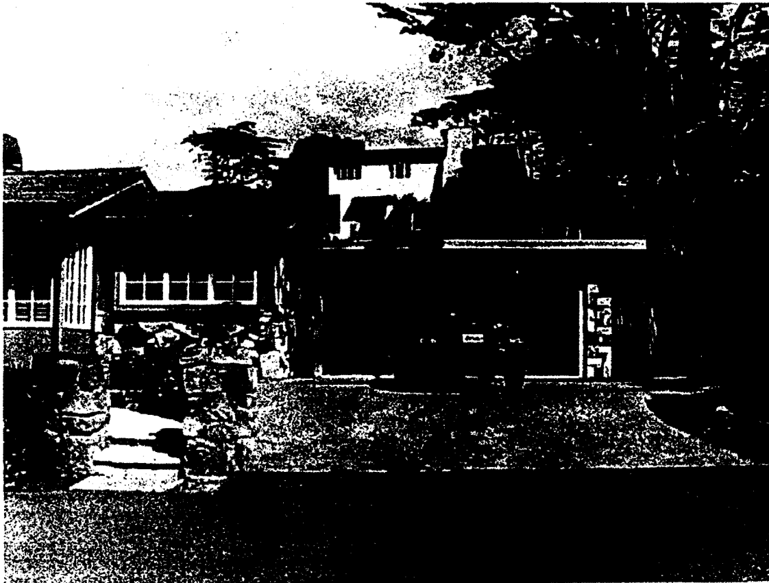
Photo 2. Continuing view of Bertuccio residence as seen from Scenic Road. This is the south wing of the structure.
