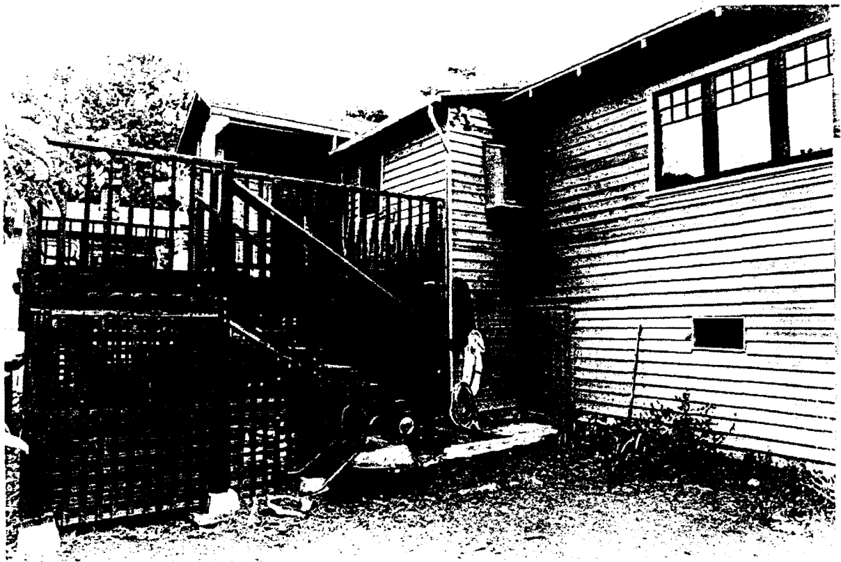
Photo 2. Rear view of existing structure and decking.
