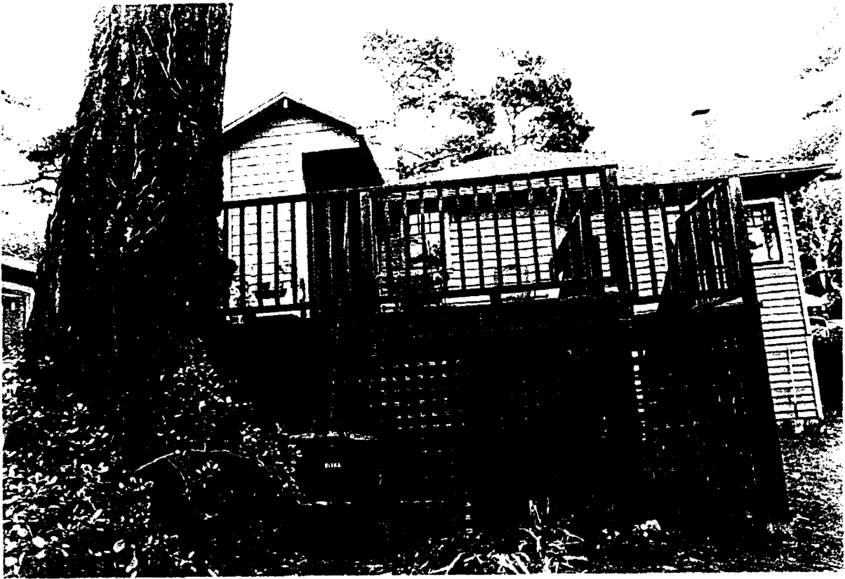
Photo 1. Rear view of existing structure shows large pine, decking, and slope of the lot.
