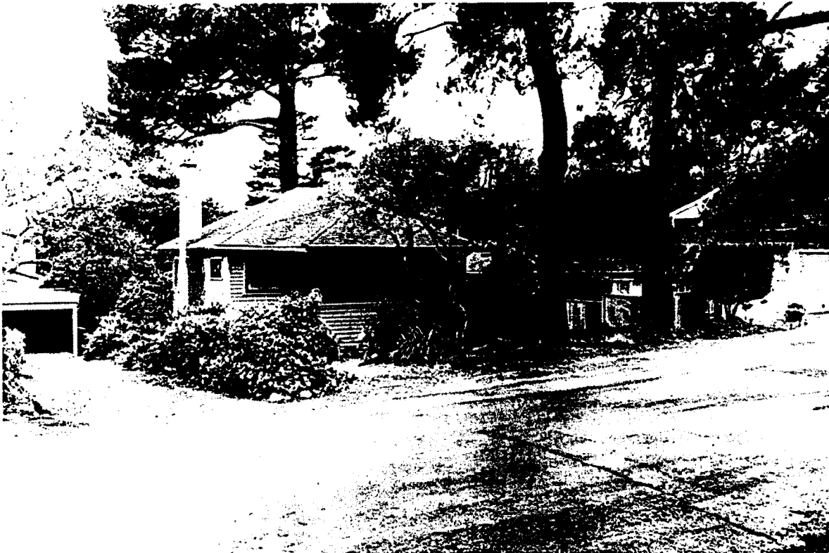
Photo 2. View of existing structure and site characteristics.
