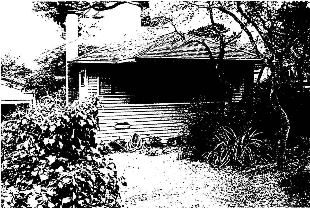
Photo 1. View of existing structure and parking pad along Lincoln.
