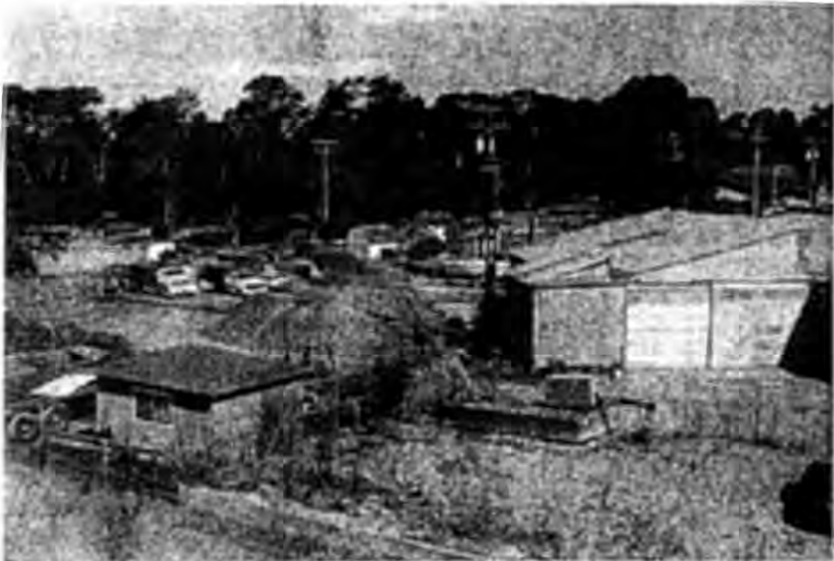
Photo 3. View of existing mill building and fenced storage areas. View looking toward Sunset Drive from southwestern property boundary.
