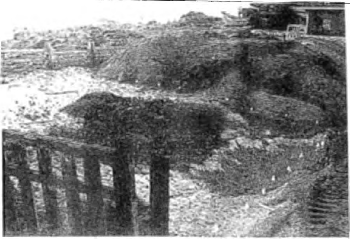
LOOKING SOUTH ONTO MILLER'S PROPERTY FROM SUNSET DRIVE
