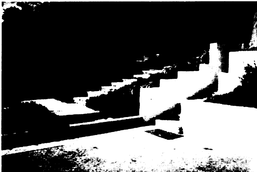
Photo Above: Lower end of stairway from Lot 1 to E. Sea Level Drive & top of stairway from E. Sea Level Drive down to beach
