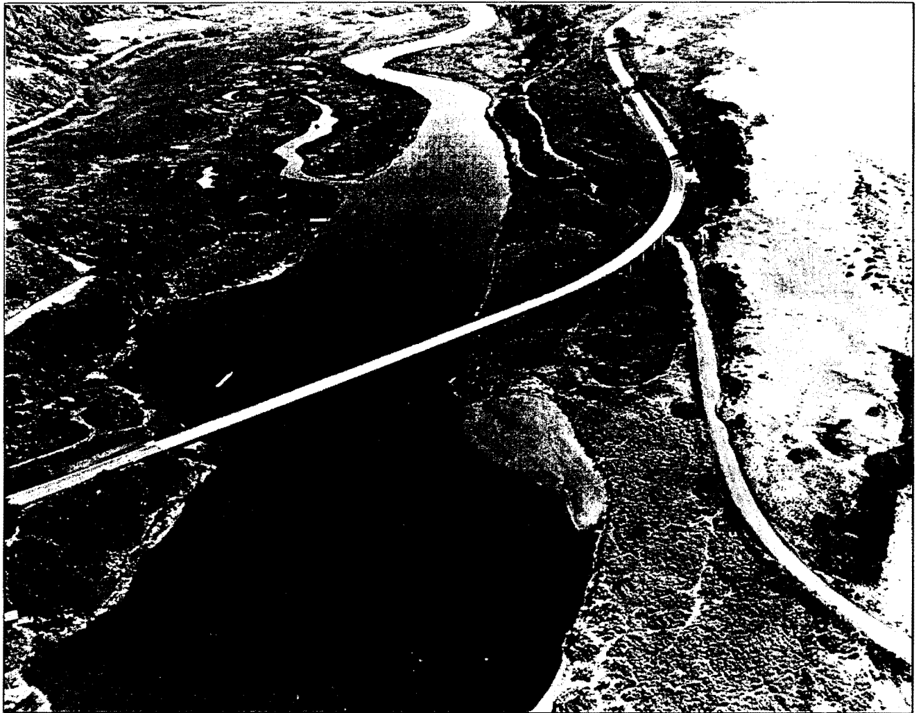
Ten Mile River Estuary and Route 1 Bridge. View towards the southeast
