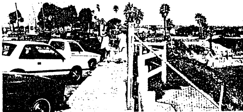
INAPPROPRIATE PARKING LOCATION PUSHES WALKWAY AGAINST HAZARDOUS BLUFF EDGE REQUIRING EXTENSIVE FENCING
