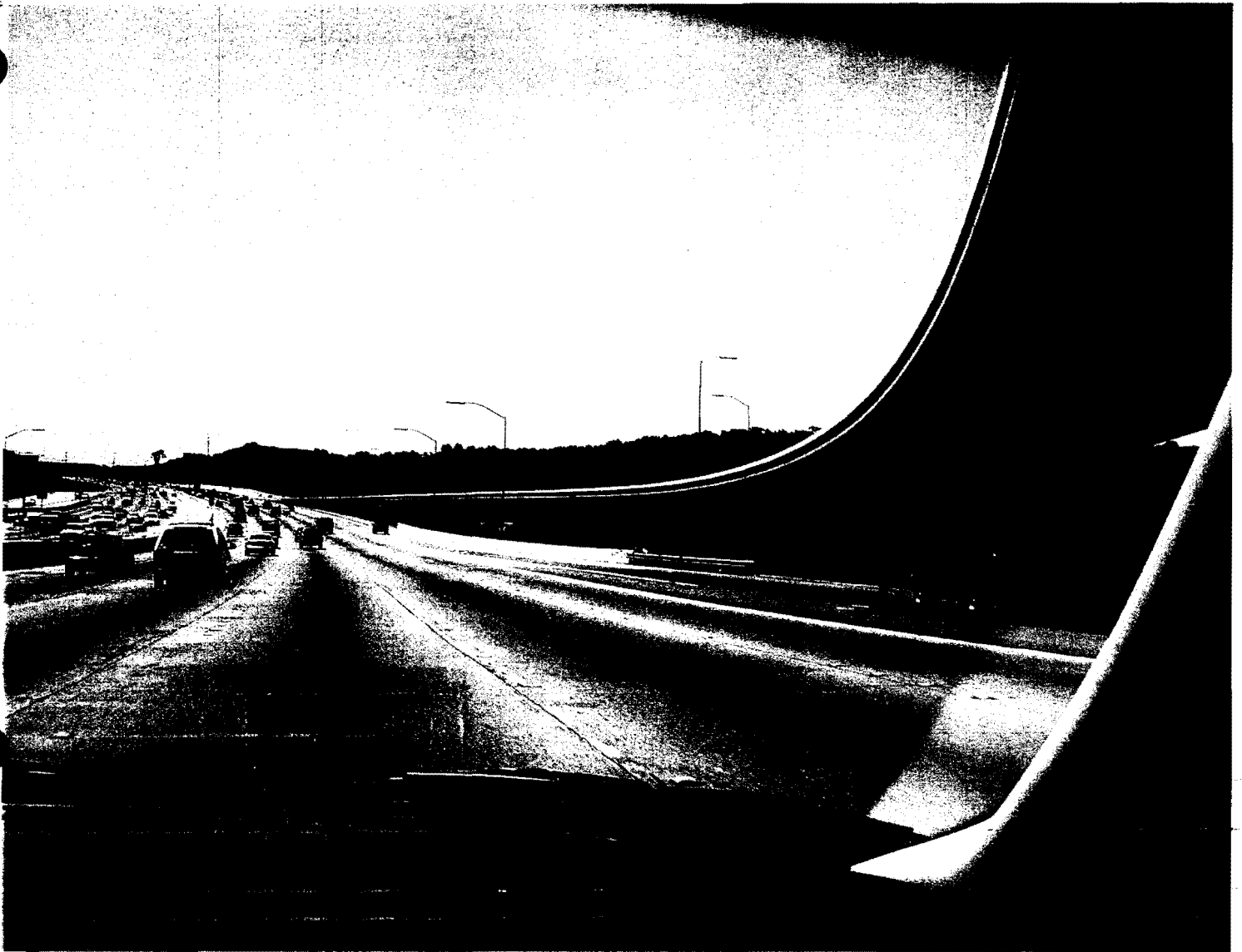
Location of proposed right shoulder concrete barrier for wildlife crossing adjacent to Carmel Valley Road on ramp to southbound I-5.
