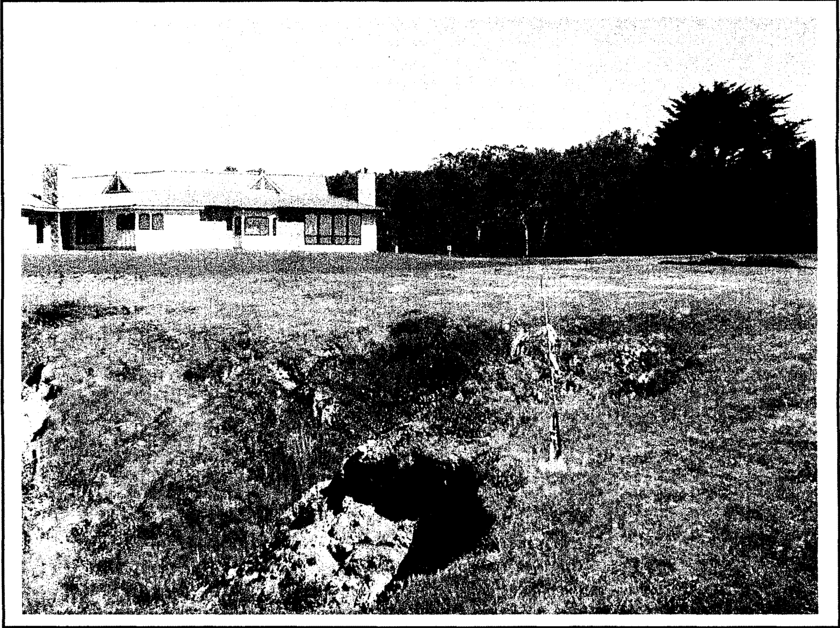
FIGURE 4: Proximity of residence to gradually eroding Coastal Bluff.
