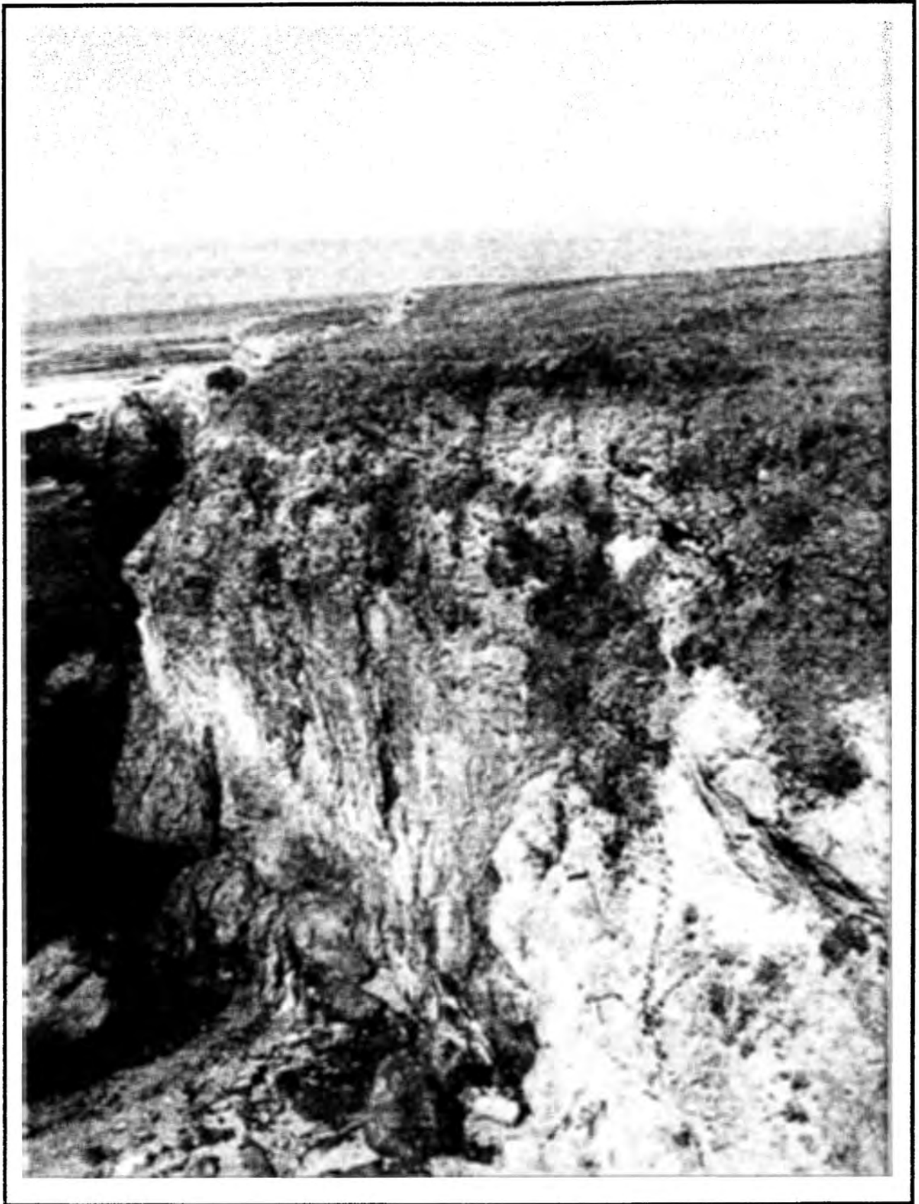
FIGURE 2: Coastal Bluff showing exposed bedrock on the bluff face.
