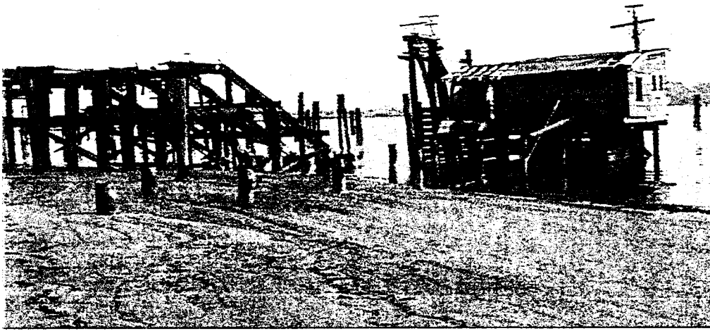
Photo #1 Southern end of Site, Log Ramp and Pumphouse
