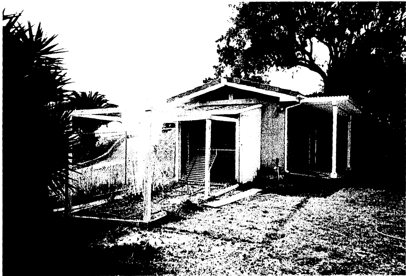
Photo 3. Storage barn on lower level. The applicants propose to expand and convert the storage barn into a guesthouse. The top of the failed slope restored by Caltrans is in the background, behind the chain link fence. View is to the southwest.
