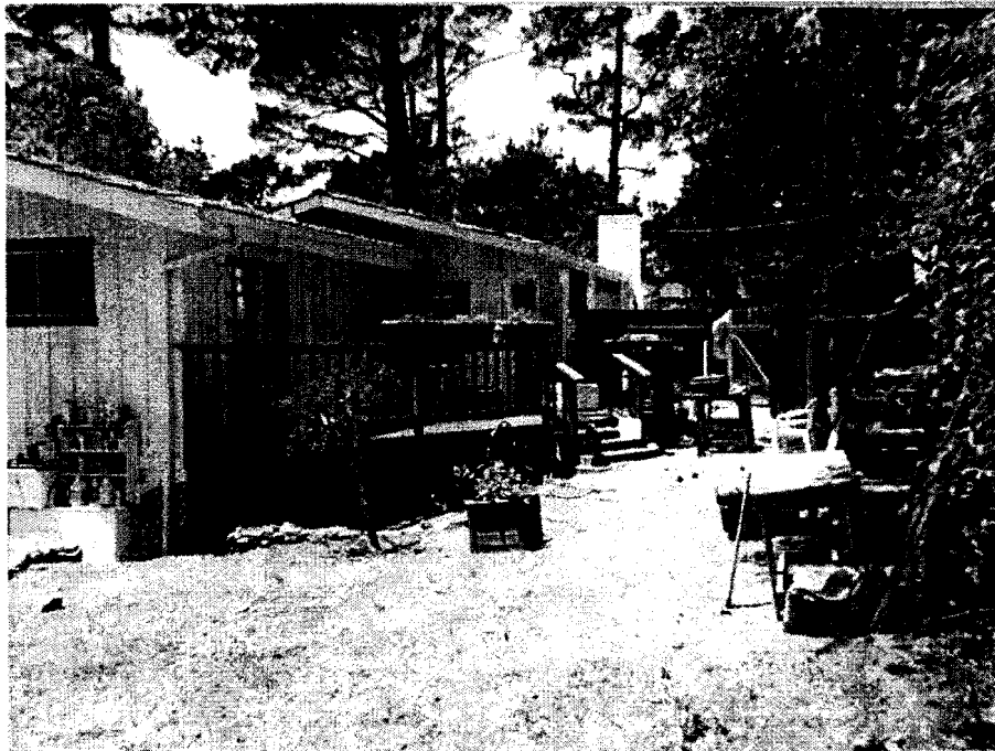
Photo of existing house from the east (rear yard).
