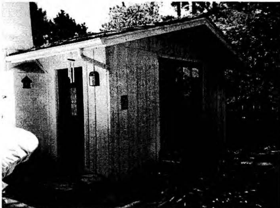
Close-up view of the entry to the existing structure.
