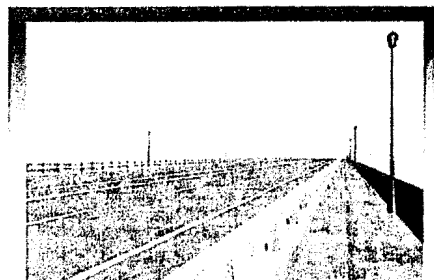
The Type 80 Rail is a concrete rail, similar to the Type 80SW, but is placed on the inside of the bridge sidewalk (between traffic and pedestrians).
