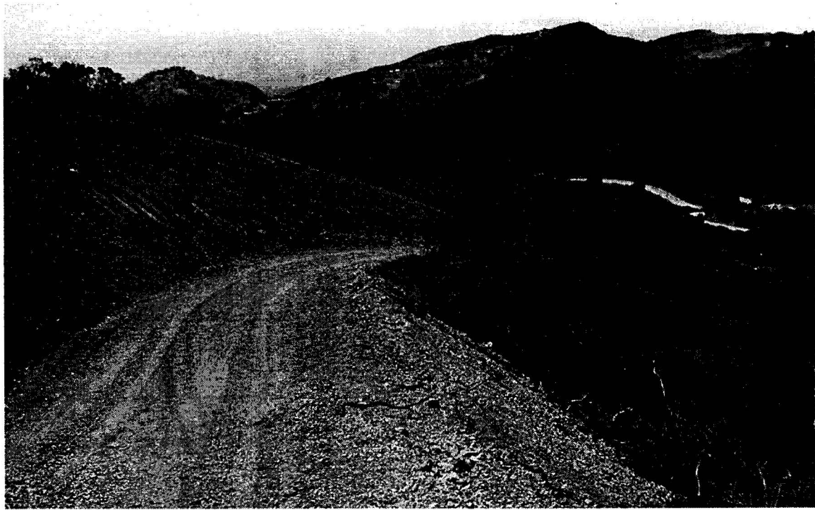
Photograph 2. View looking generally south on subject property showing newly graded road and steep slope that has been cleared of vegetation.
