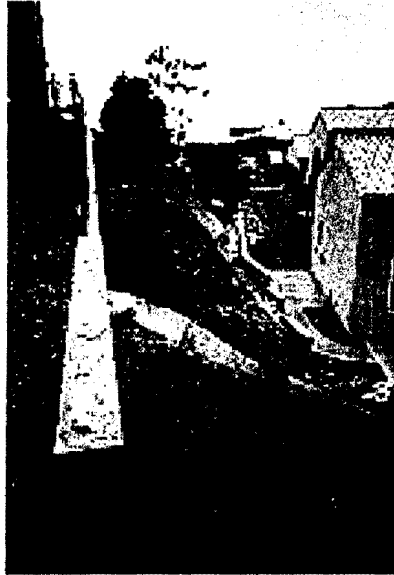
Photo 4: Retaining wall on southern property line, looking east.
