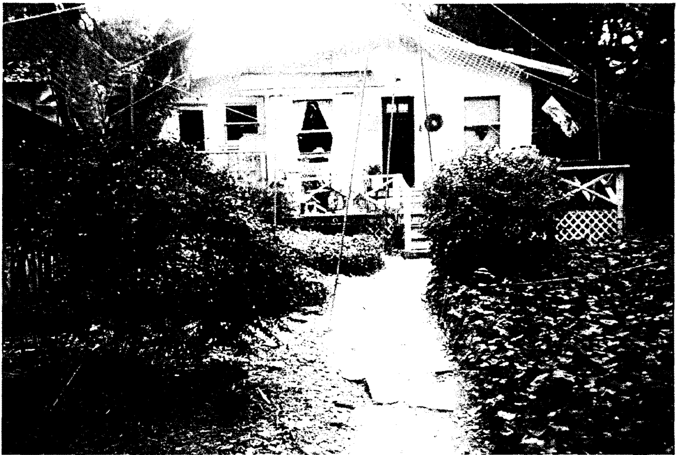
Photo 1. View of existing structure from Lincoln Street
