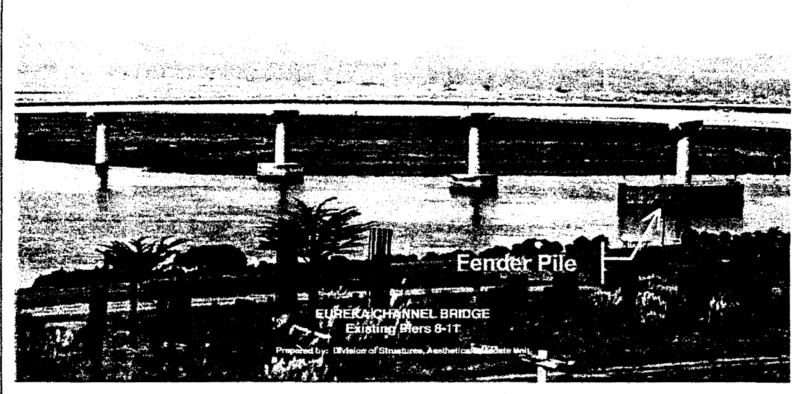
View of Existing Eureka Channel Bridge Facing North
