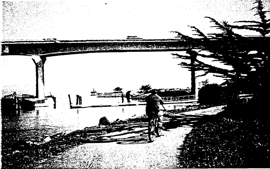
Existing Eureka Channel Bridge Facing East
