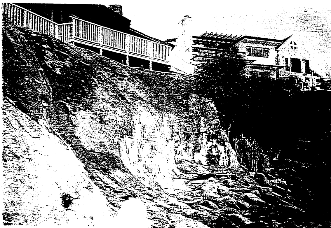
Figure 6. Gunitite covered bluff from beach level. The undermined area is located at the base of the bluff to the left of the vegetation at the end of the wall. The sea-cave is located behind the vegetation near the base of the bluff.
