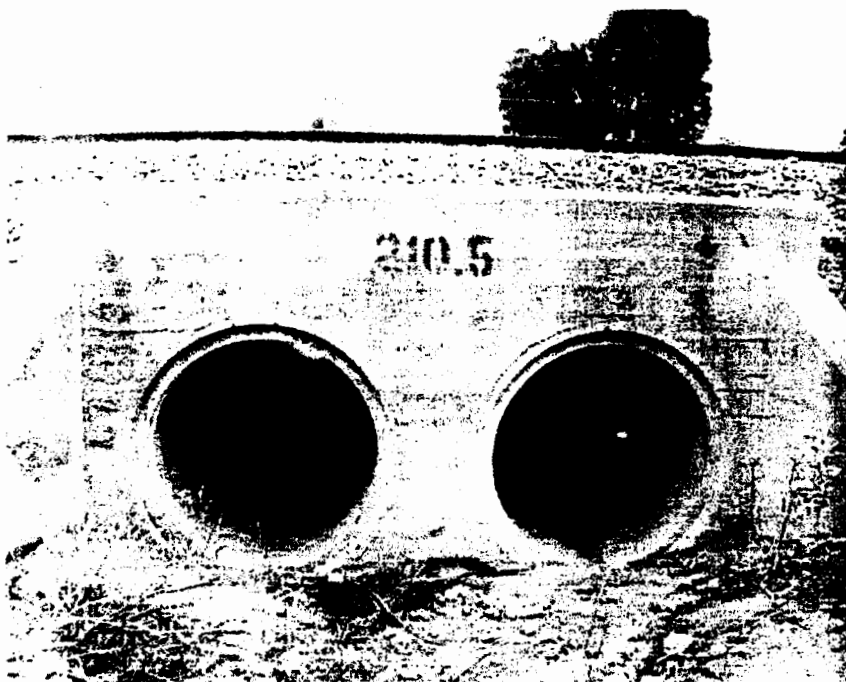
View of east face of Culvert MP 210.5 (Station 721+22.3).
