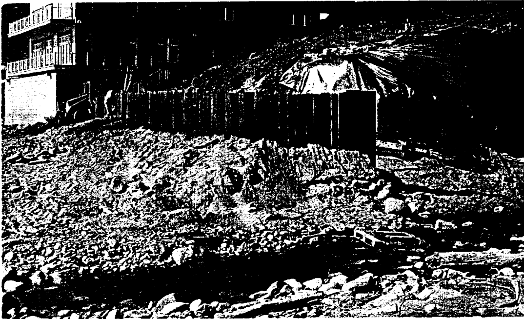
The seawall/planter and Little Sycamore Canyon Creek under construction viewed from the beach on March 17, 2003
