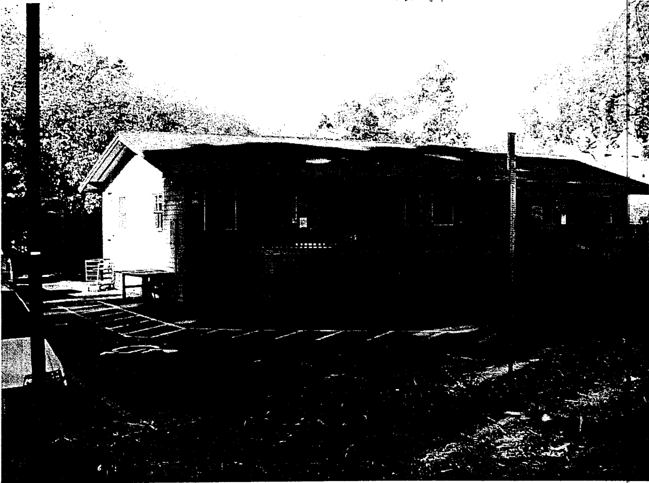
Figure 2: Love Lab Trailer Existing Location
