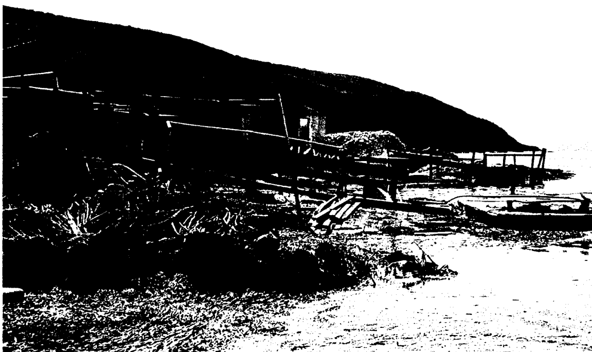
Oyster cultivation equipment and refuse stored or discarded in the tidal zone, and unpermitted commercial structures in the background.
