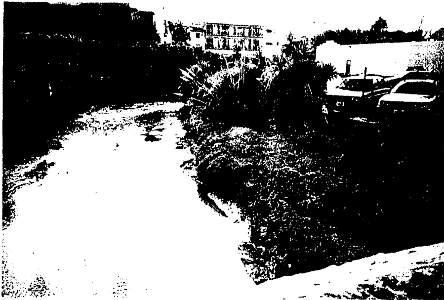
Photo 1 - Looking upstream from State Street Bridge - Feb 17, 1998
