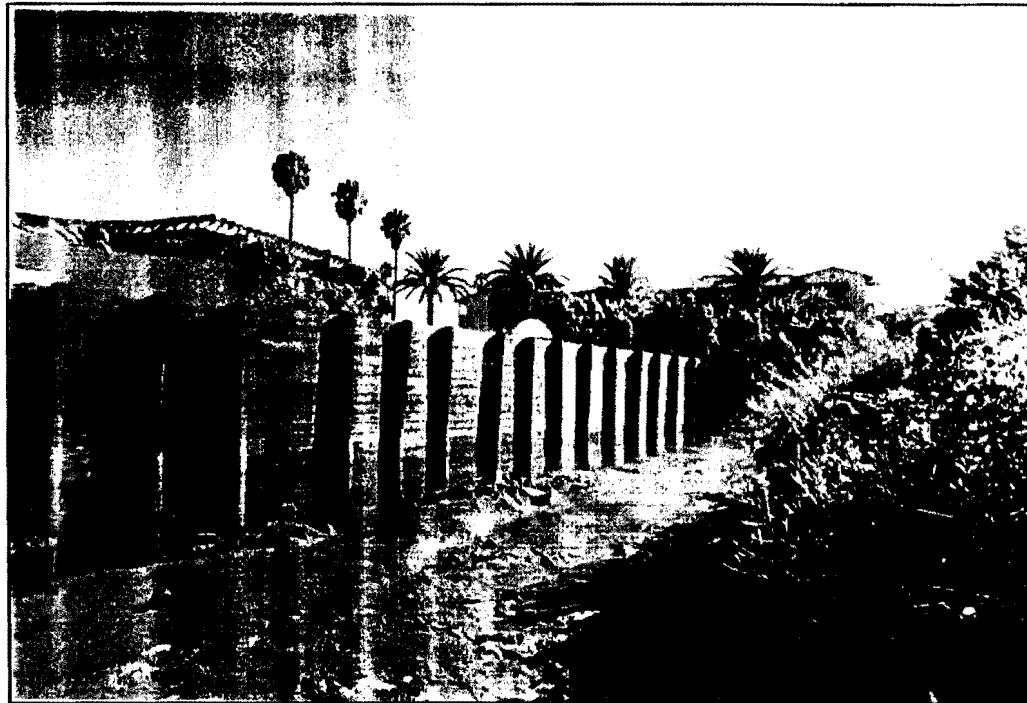
Replacement bulkhead during low flow period in 1995
