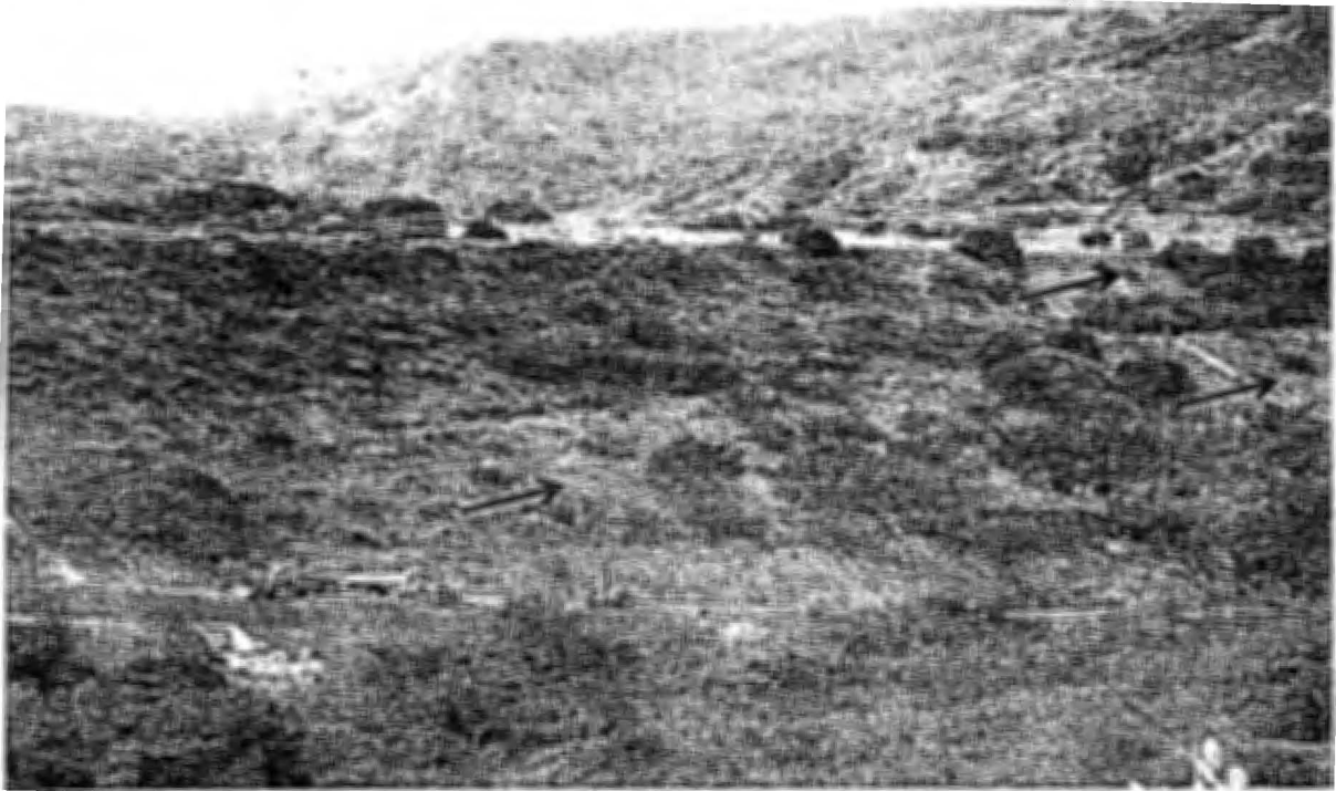
Photo 3: The easterly facing fill slope on Lot 1 above the bridge that crosses onto Lot 2 is also adequately revegetated except in a few areas where selective broadcast- and contour seeding shall be done as indicated by the red arrows. The access road across Lot 1 and the outlet for the bench drains of Lot 1 are shown in the lower section of the photograph.
