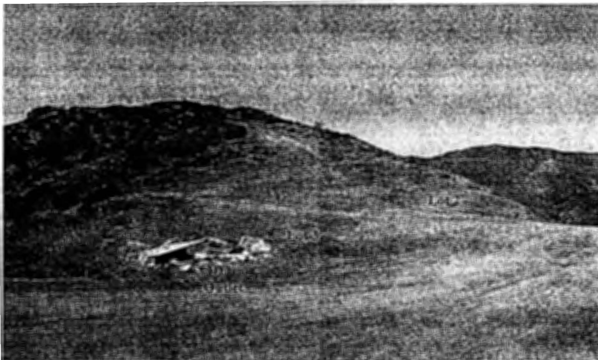
Photo 15: As is evident from this photograph, this fine-graded northerly facing cut slope and the surveyor's access road to the knoll need to be revegetated. This road is the approximate boundary between Lots 2 and 3 (compare with Photo 10). The undermined outlet dissipater should be repaired.
