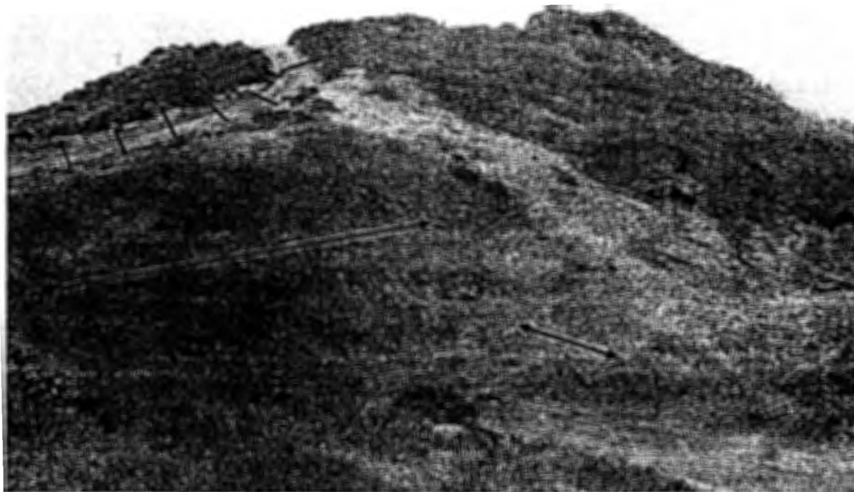
Photo 10: This northeasterly facing 'bedrock' cut slope on Lot 2 presents a special challenge. It should receive supplemental watering during the first year seedling establishment period.
