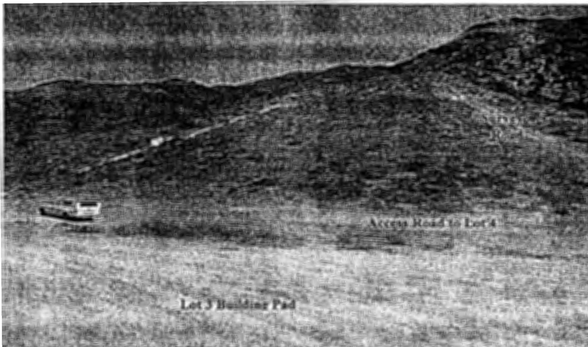
Photo 14: This view is looking northerly from the building pad of Lot 3 across the access road to Lot 4. Selective restorative broadcast- and contour- seeding should be carried out on the easterly facing bench drain-dissected cut slope and more intensive restoration contouring along the access road cut into the hillside by the 4-wheel-drive vehicles of the surveying crew.
