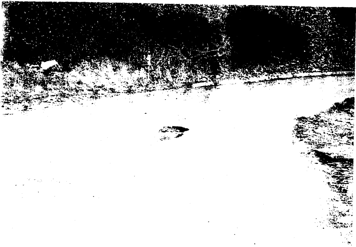
HOLES IN ACCESS ROAD DUE TO SPRING ACTIVITY 1 ↑ 2 ↓
