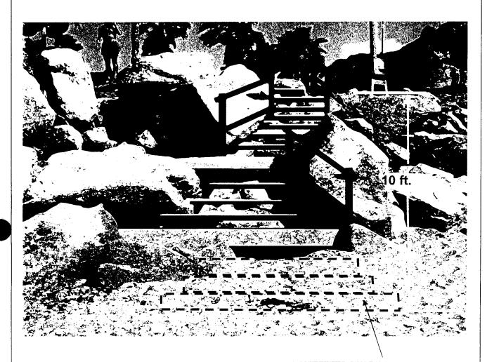
Subterranean steps. The grade of the beach changes frequently. The proposed design includes a section of steps which appears below grade in the photo rendering above.
