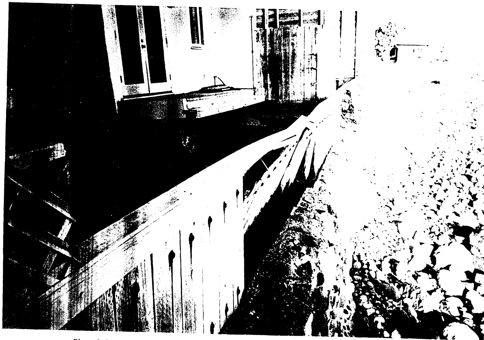
Photo 3. Damaged seawall, with wood deck and septic area behind. View is to the northeast.
