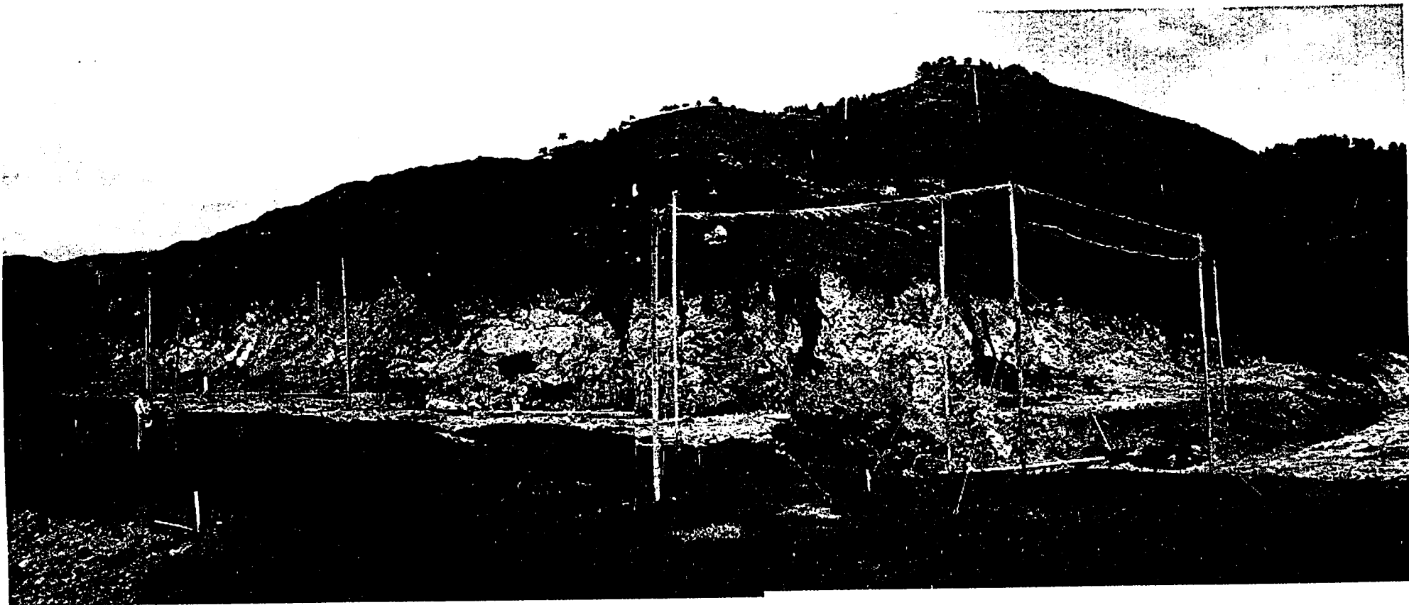
Photo 3. Project staking, looking east at cut face; theater/media area is shown staked on left side of photo. Photo shows excavated building pad and cut face, and access road on right.
