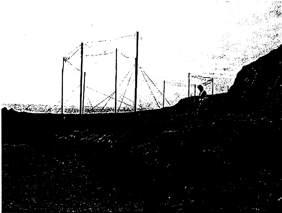
Photo 2. Project staking, looking north; theater/media area is staked at rightmost of photo (against bluff). Photo shows excavated building pad and cut face on right.
