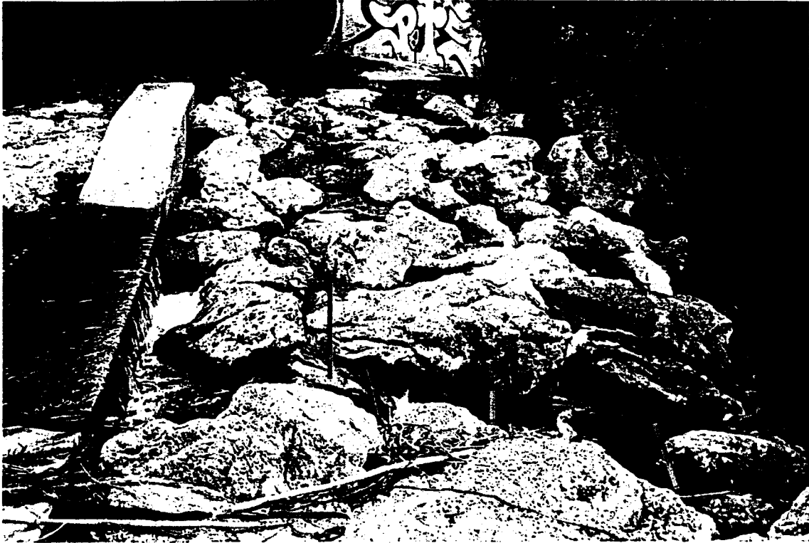
Photograph No. 9. Location of proposed concrete weirs to create small jump pools.
