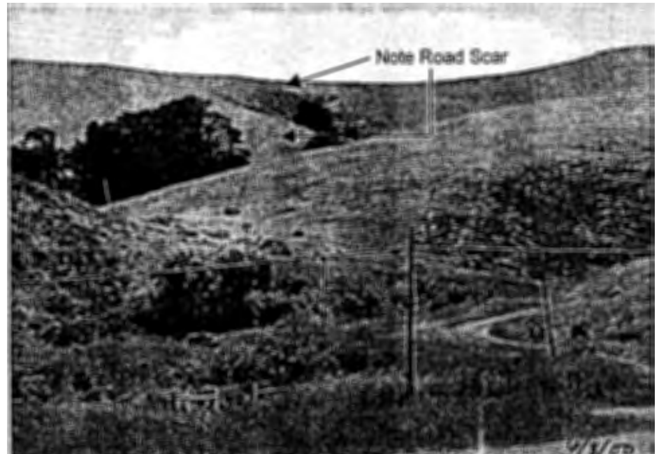
Existing Entrance & Access Road as viewed from Hwy 1
