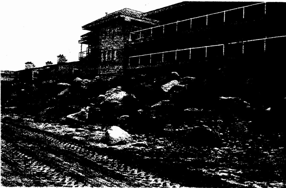
Photograph 2. Subject revetment June 11, 2003, looking north.
