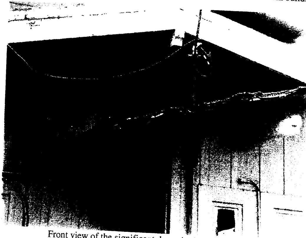
View of severe decay and poor support to the roof pop-out area of the main building.
