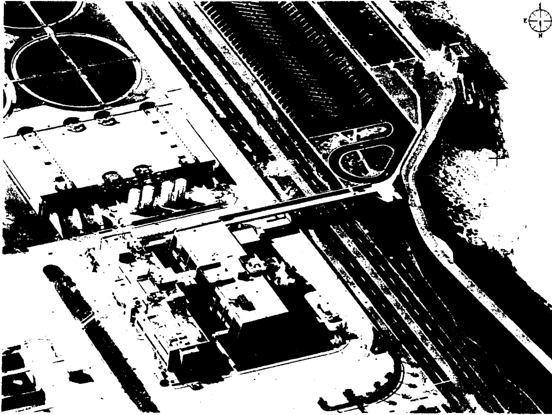
Vista Del Mar bridge connects the Hyperion Treatment Plant to a County of Los Angeles parking lot across Vista Del Mar.
