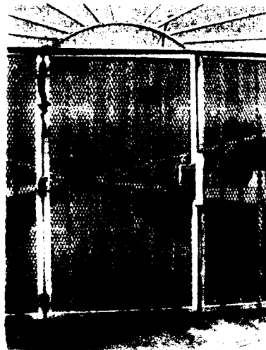
There is a locked gate limiting access from the beach side to Hyperion Treatment Plant.
