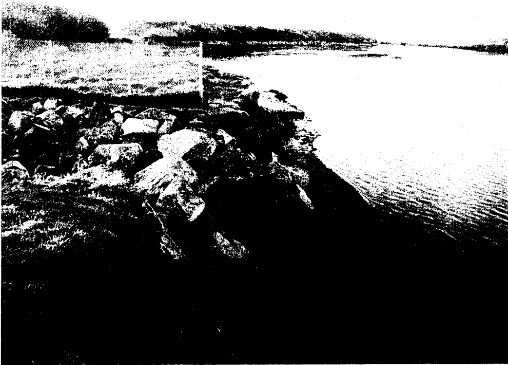
Looking Upstream at Outfall Outlet (February 10, 2005)
