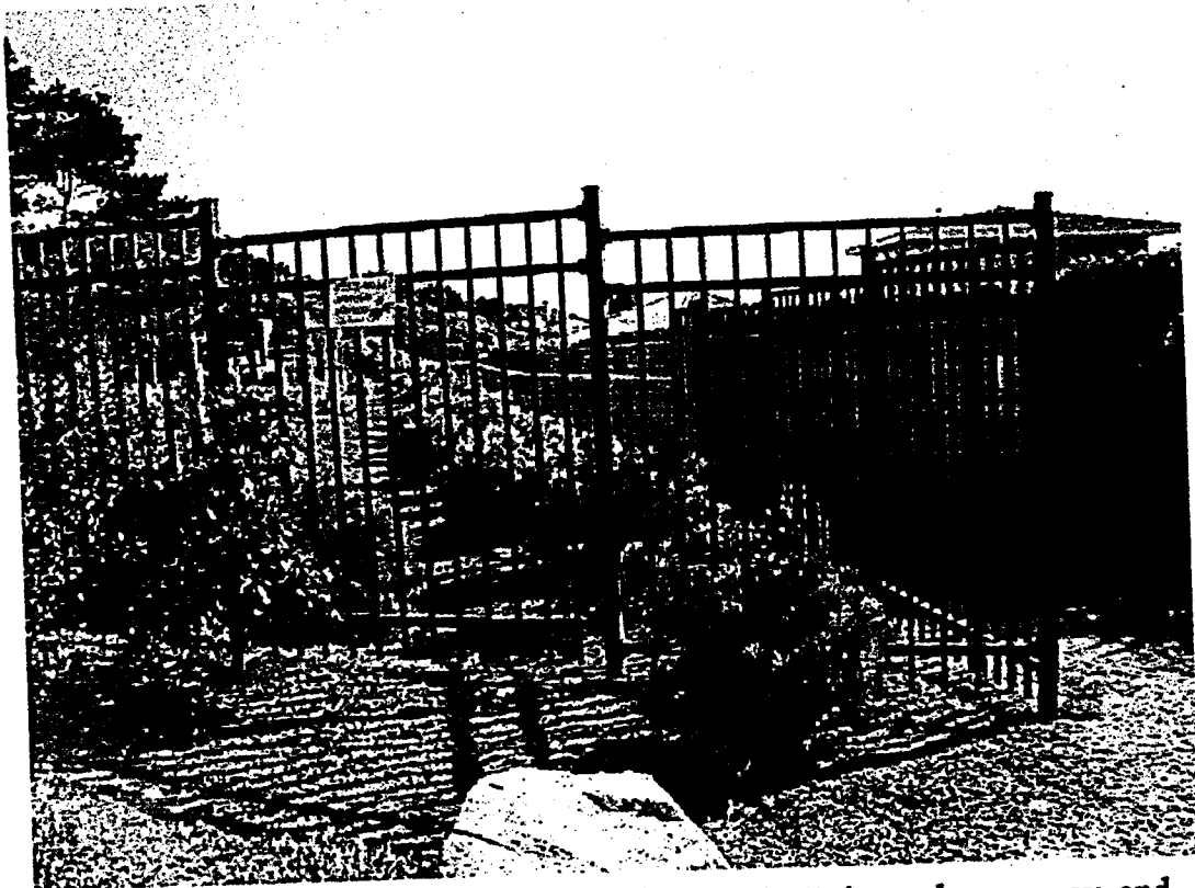
Photo 3. Six-foot high metal fence fronting Yankee Point Drive and accessway, and four-foot high wood-and-wire fence along accessway (on Parcel APN 243-161-017).
