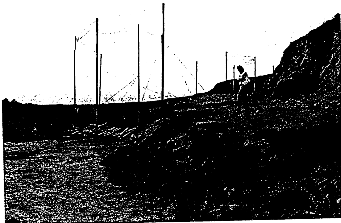
Photo 2. Project staking, looking north; theater/media area is staked at rightmost of photo (against bluff). Photo shows excavated building pad and cut face on right.
