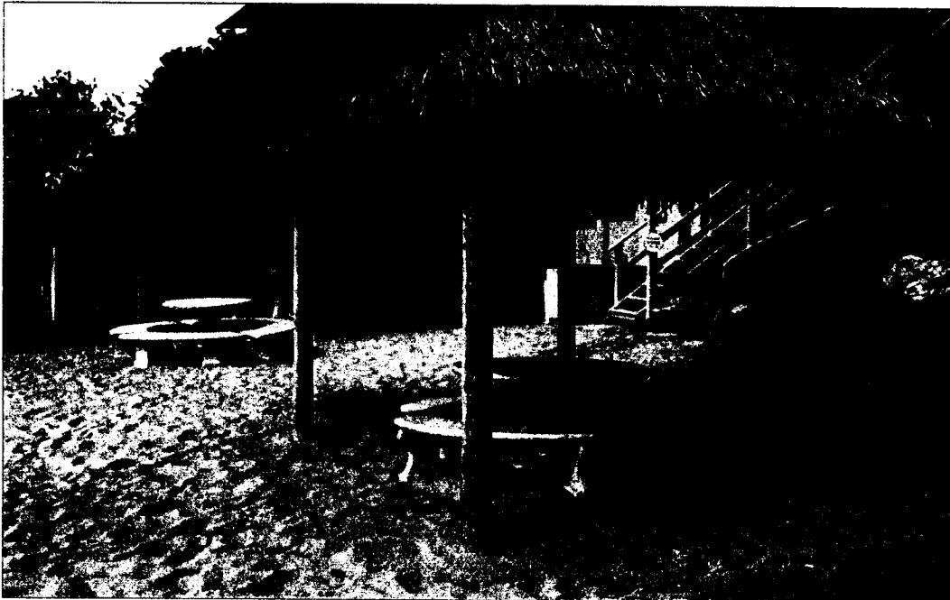
Exhibit 2d. February 2004 photograph of unpermitted shed, barbeque area, storage cabinets, concrete picnic tables and benches, and shade/canopy structure on subject property. Shed to the left of the stairway is set into graded toe of bluff; vegetation has been removed from toe of bluff to the right of the stairway.
