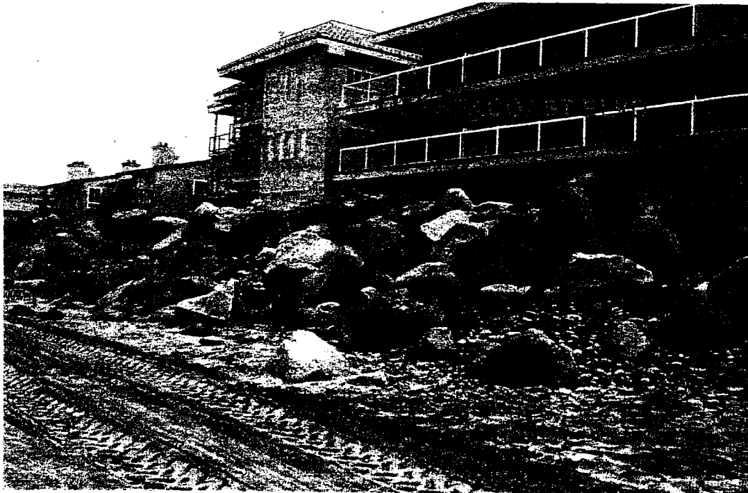
Photograph 2. Subject revetment June 11, 2003, looking north.
