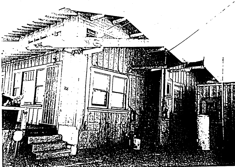
Photograph #8 706 Manhattan Court "The Turquoise House" East Elevation
