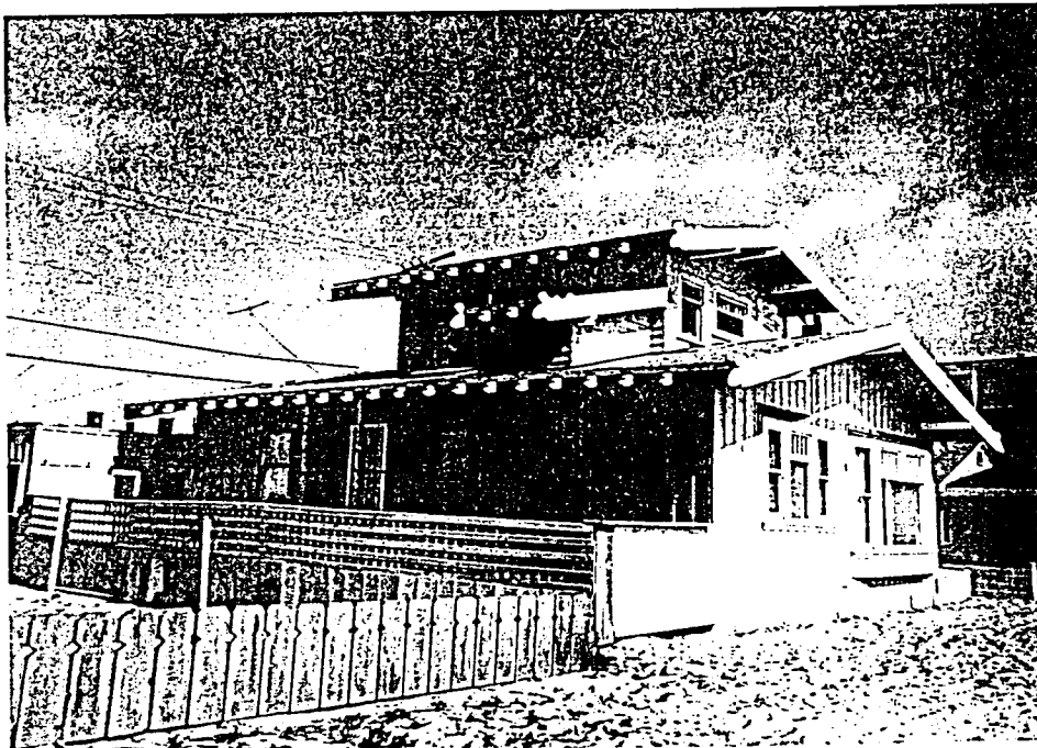
Photograph #2 706 Manhattan Court "The Turquoise House" North & West Elevations View Facing South
