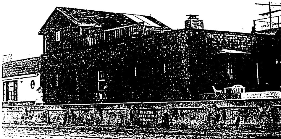
Building #6 702 Whiting Court "Bungalow" Identified In Mission Beach Survey (1997)
