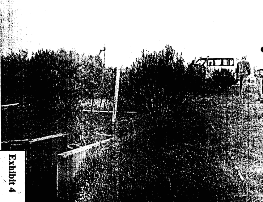
Seasonal wetland area to be temporarily disturbed for replacement/installation of drain pipes.
