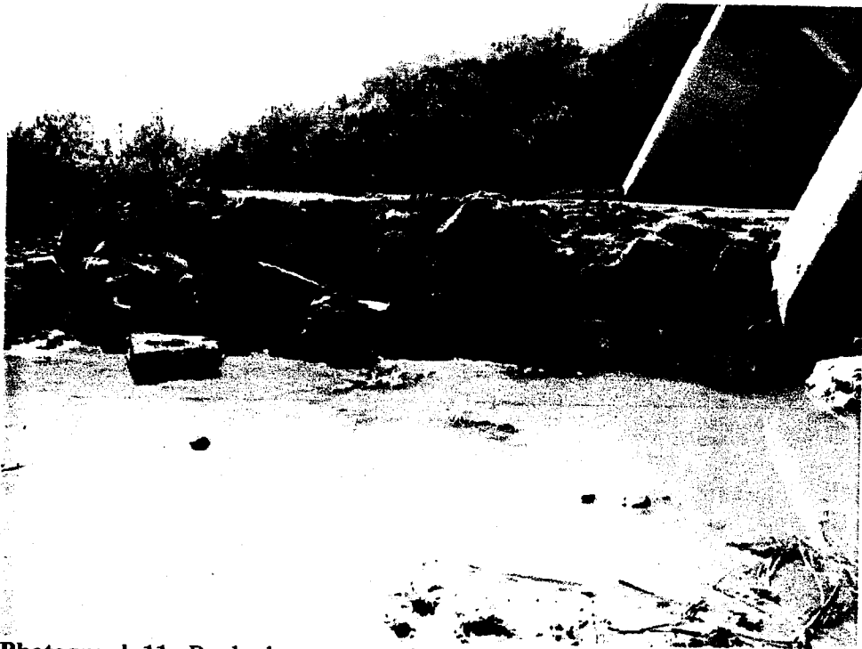
Photograph 11. Rock placement on downstream side of bridge pier (6 April 2005)
