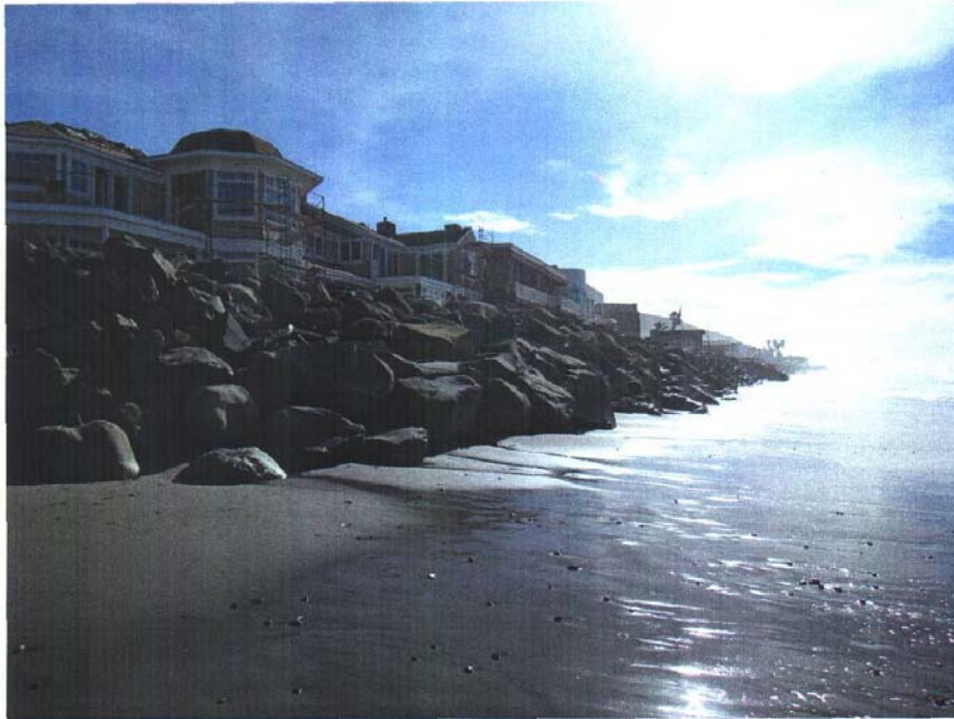
Looking Northeast at Existing Revetment: Applicant's Residence Located to Left.
