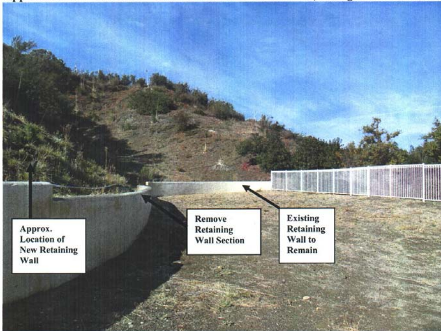
View to Northwest of Flat Pad Area Behind Residence Where Pool, Pool Enclosure and Pool/Guest House are Proposed. Existing Retaining Wall to be Removed & New Retaining Wall to be Constructed to Left.
