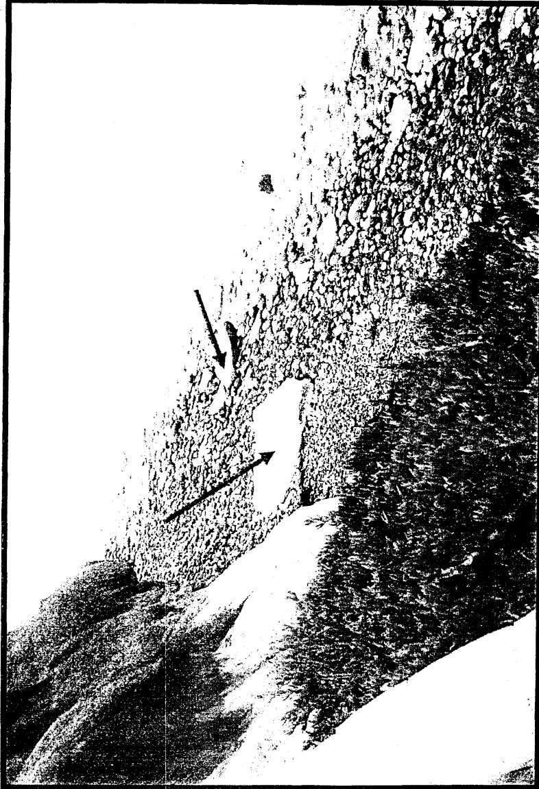
Figure 6 Several large slabs of gunite from erosion control at subject property. This failure occurred after the 2002 aerial photo (Fig 3).
