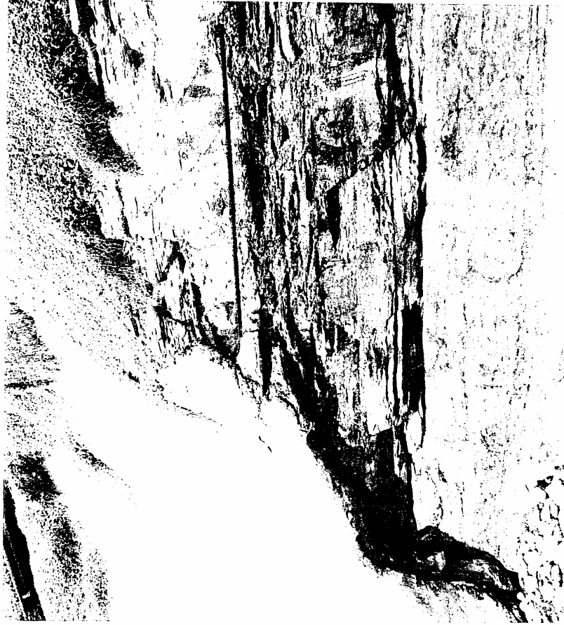
Figure 8 Seepage ( below red line) and fractured rock at southern edge of gunitite erosion control at subject residence
