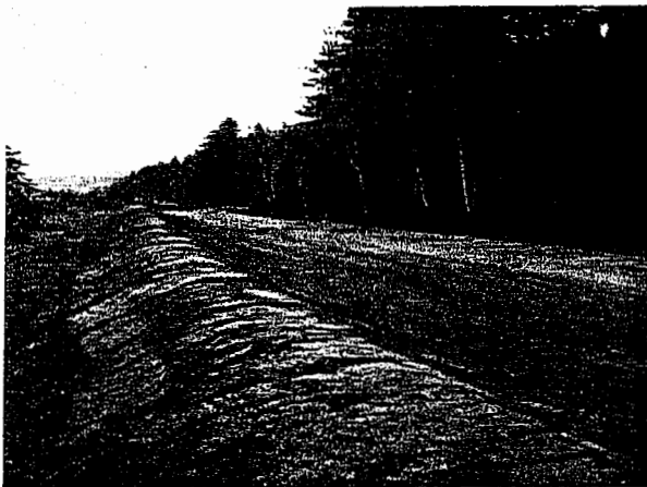
Figure 14. Upper dike section that was set back to create new floodplain.
