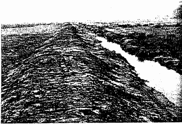
Figure 13. Lower section of reconstructed dike adjacent to the salt marsh. Wetland plant material was salvaged and replaced back into the channel during the dredging operation.
