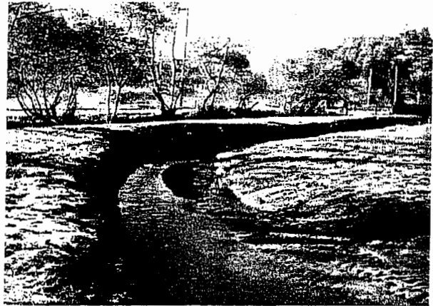
Figure 11. Newly reconstructed upstream channel reach with habitat structure and small gravel deposit from late-October rainstorm.
