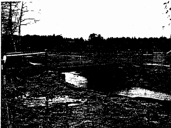
Figure 17. A bridge was installed to replace the culvert and provide cattle access to the north side of the pasture.
