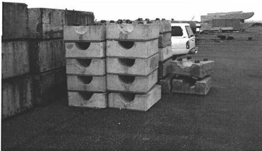
Photo 1: Self fabricated 1,500 lbs concrete weights to submerge the pipeline.
