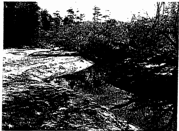
Figure 12. Newly reconstructed lower slough channel that replaced the straightened, aggraded section and eliminated 90-degree bends.
