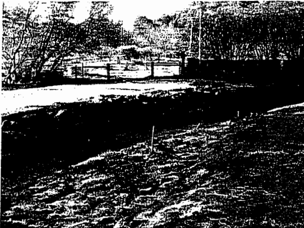
Figure 16. Bank RSP and grade control were installed to protect the Eureka waterline crossing.
