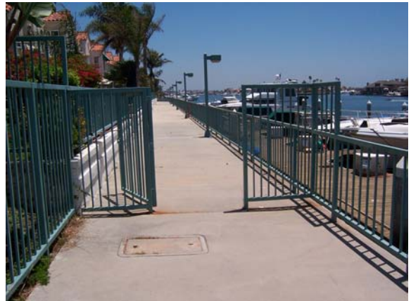
Public walkway along bulkhead.
